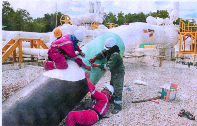
Taking no chances: Workers installing a special adhesive on a gas pipe to prevent gas leakage as a step to face the expected high-tide phenomenon in Klang. — Bernama
